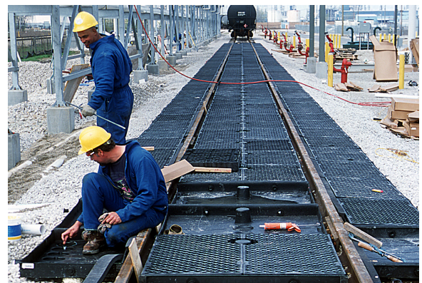
Modular Design Center and Side Pans are 53.5" long; containment areas can be easily assembled to any length desired.
